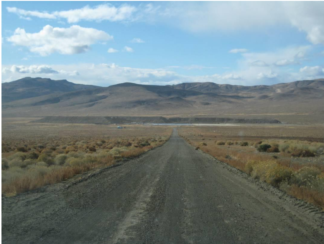
Figure 5.2 Photograph Showing Physiography of Relief Canyon Area (Lacana/Pegasus Heaps in middle ground)
